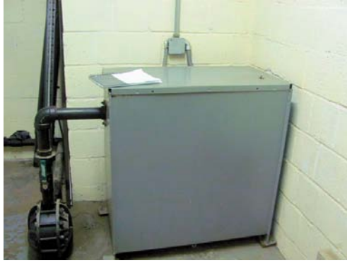
Elevator control unit
