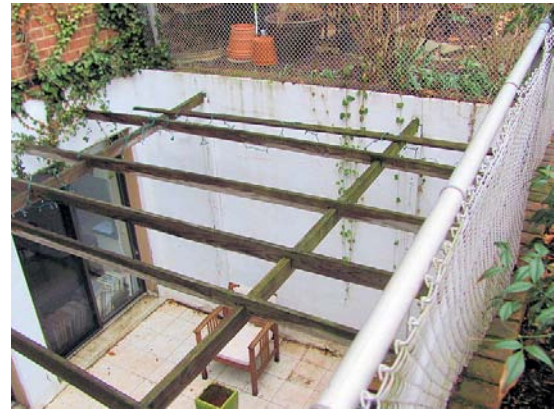
Block retaining wall at patio area
