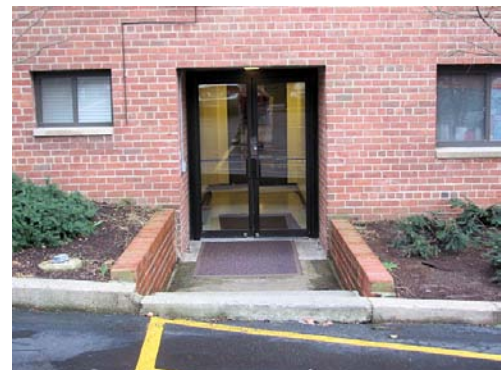
Side entrance doors
