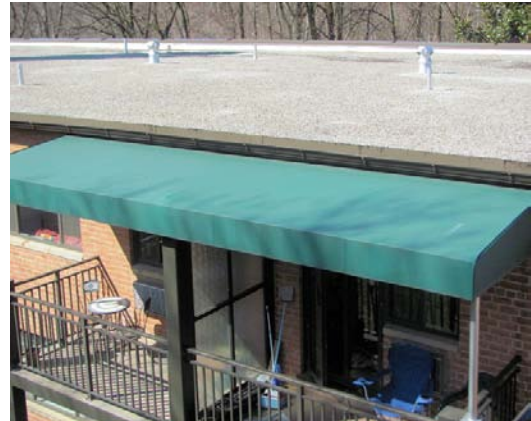
Top view of balcony canopy
