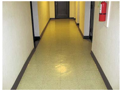
Vinyl tile at rear corridor
