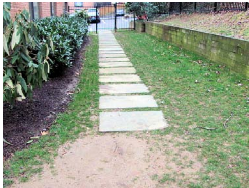
Wood retaining wall and slate stepping stone pavers at rear of building
