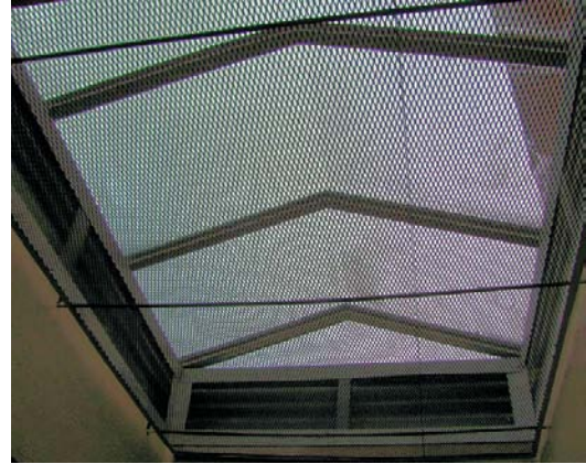
View of skylight from stairwell
