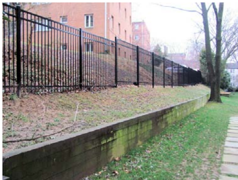
Aluminum fence at rear of building
