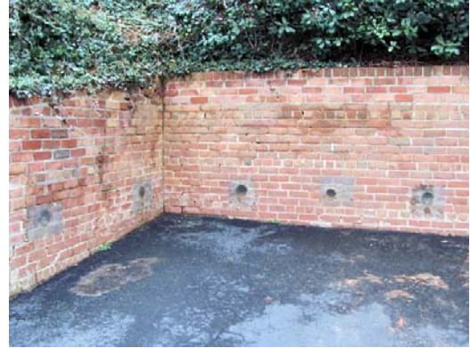
Brick wall at rear property line with top 4 courses repaired
