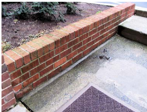
Brick walls at side entrance
