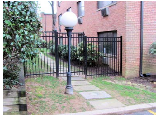
Typical pole light scheduled for replacement
