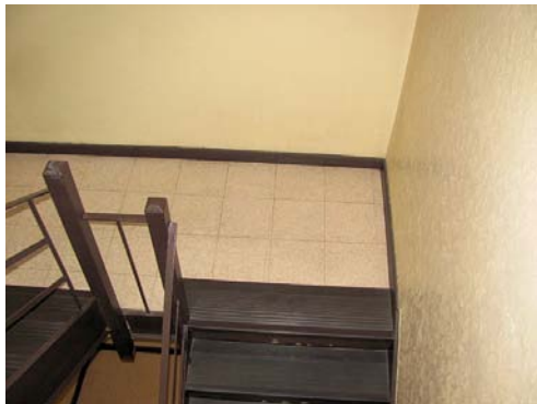
Typical stairway tile, treads and rails
