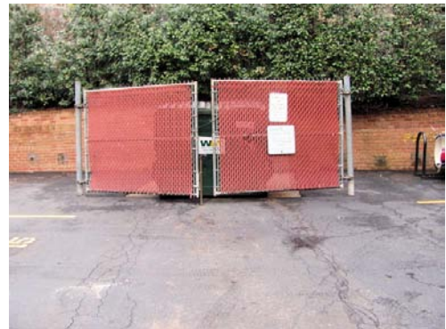
Trash corral chain link fence gates
