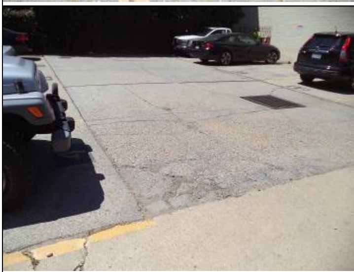
Photo #30: One section of the rear concrete parking is damaged, and should be scheduled for replacement.
