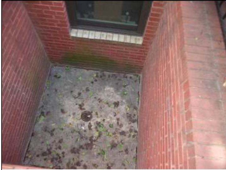
Photo #7: Joints between concrete and brick walls. This should be sealed with caulking, which would prevent damages to the subbase materials.
