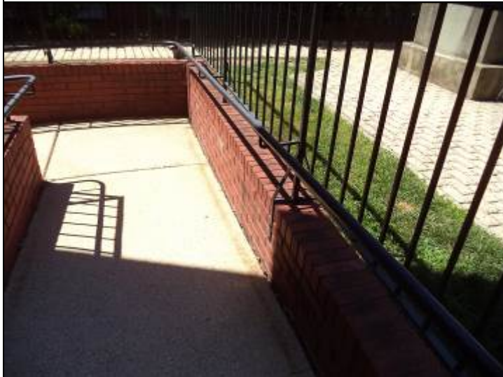
Photo #17: Joints between concrete and brick walls. This should be sealed with caulking, which would prevent damages to the subbase materials.
