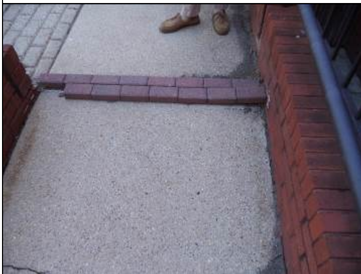
Photo #18: At the rear of 11 th Street, the building has brick installed to create a dam. This presents a hazardous condition. In this same area, the concrete walk is cracked and lifted. Consideration should be given to installing a landing at this area, which would operate as a dam and meet legal requirements as well as repair the cracked area.
