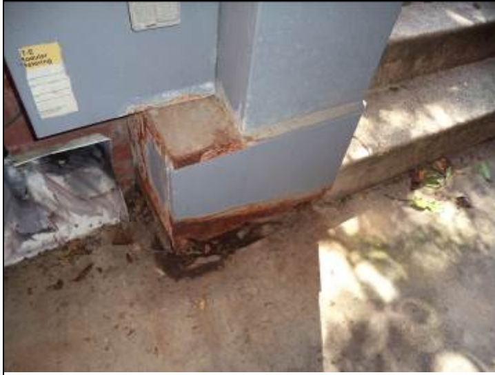
Photo #25: Some of the lower boxes for the electric service are oxidizing. Consideration should be given to having these cleaned and painted.
