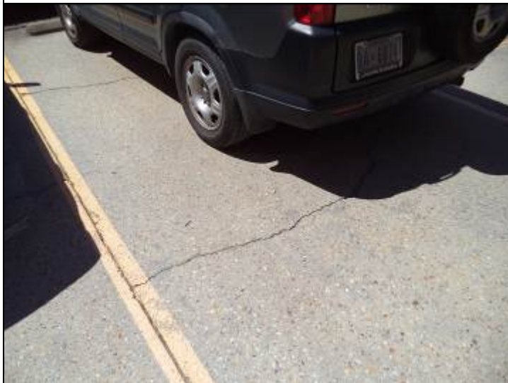
Photo #29: There are cracks in the concrete parking, which should be sealed.
