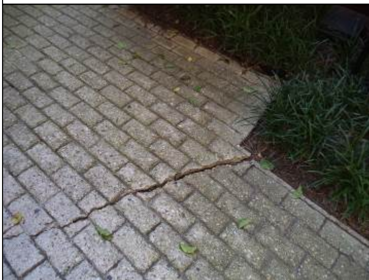
Photo #3: Outside of building 1225 there is a differential in the walk, which presents a trip hazard.
