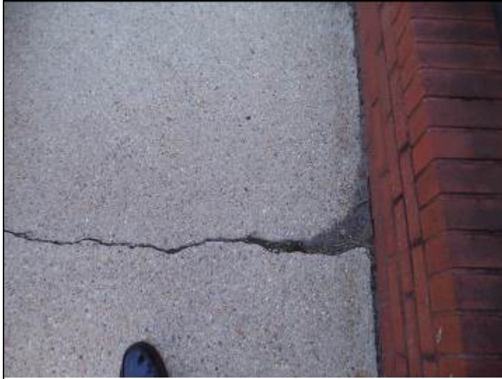
Photo #19: Cracked concrete
