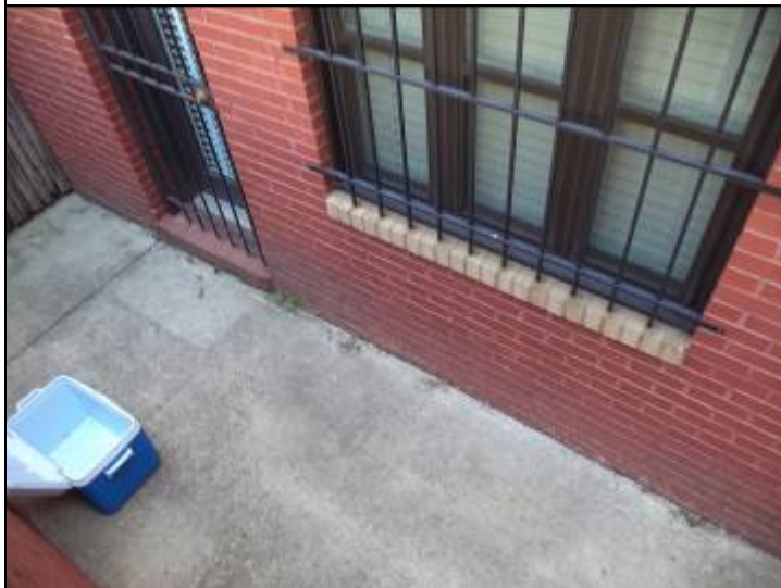
Photo #20: Joints between concrete and brick walls. This should be sealed with caulking, which would prevent damages to the subbase materials.
