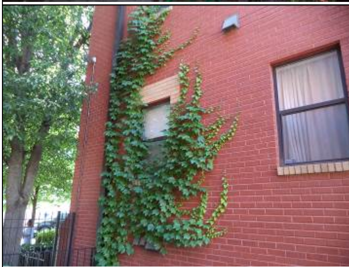
Photo #15: In some areas ivy is growing on the building, which should be prevented. Ivy will cause damages to the wall systems.
