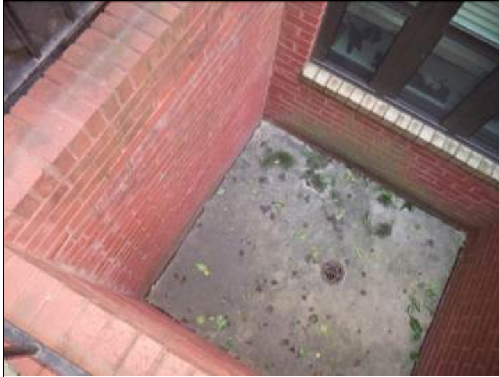
Photo #4: Joints between concrete and brick walls. This should be sealed with caulking, which would prevent damages to the subbase materials.
