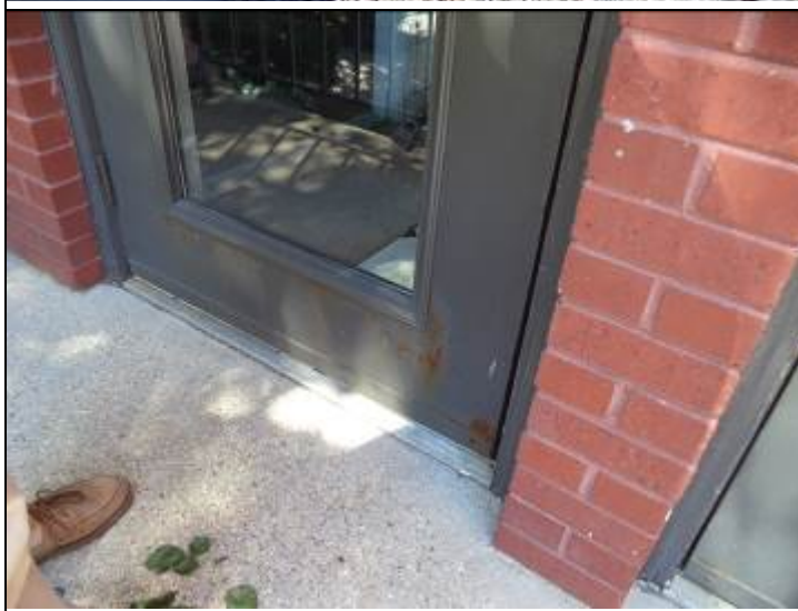
Photo #12: At the building entries on 12th Street, the doors require to be refinished.
