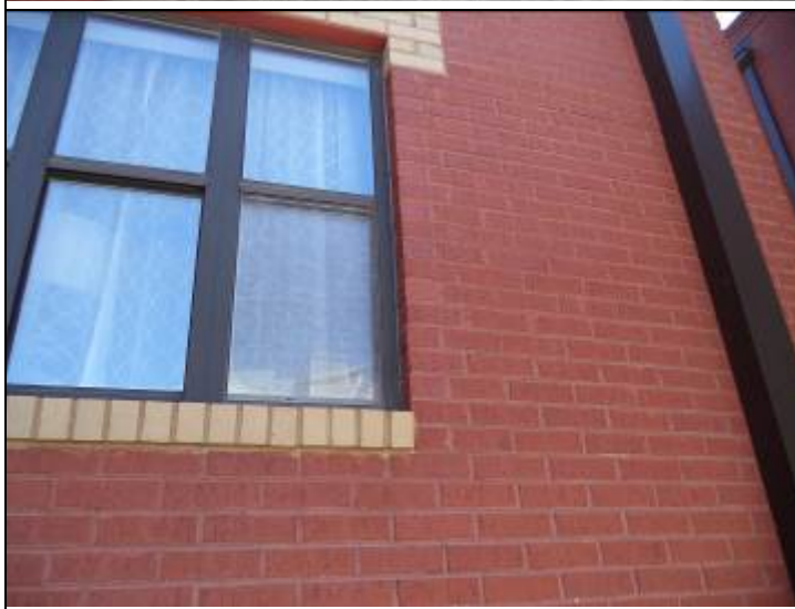
Photo #21: The caulking of the windows is deteriorated, and should be scheduled for replacement in the near future.
